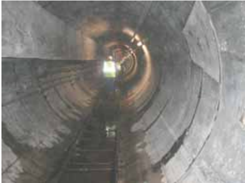
Storm water storage tunnel
