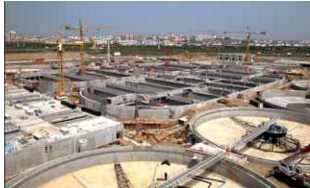
Seine amont treatment plant extension
