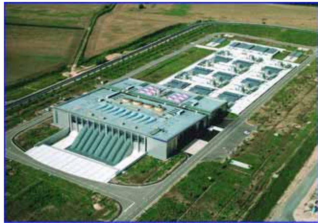
Storm water treatment plant (30 m 3 /s)
